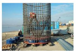
Final assembly of reinforcing cage with O-cells
