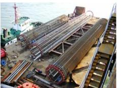
Cage sections in preparation Several lengths of reinforcing cage had to be spliced together over the bore.
