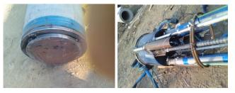
Prior to driving the first section of pile, a special shoe was inserted into the hollow section of the PHC pile and welded in place. The shoe acts like the plug of soil that forms inside the PHC pile during open-ended driving conditions but also allows for a suitable bearing surface for the base of the O-cell. The O-cell, related instrumentation and strain gauges already fixed to a reinforcing cage were inserted into the hollow centre of the PHC pile and concreted in place.
